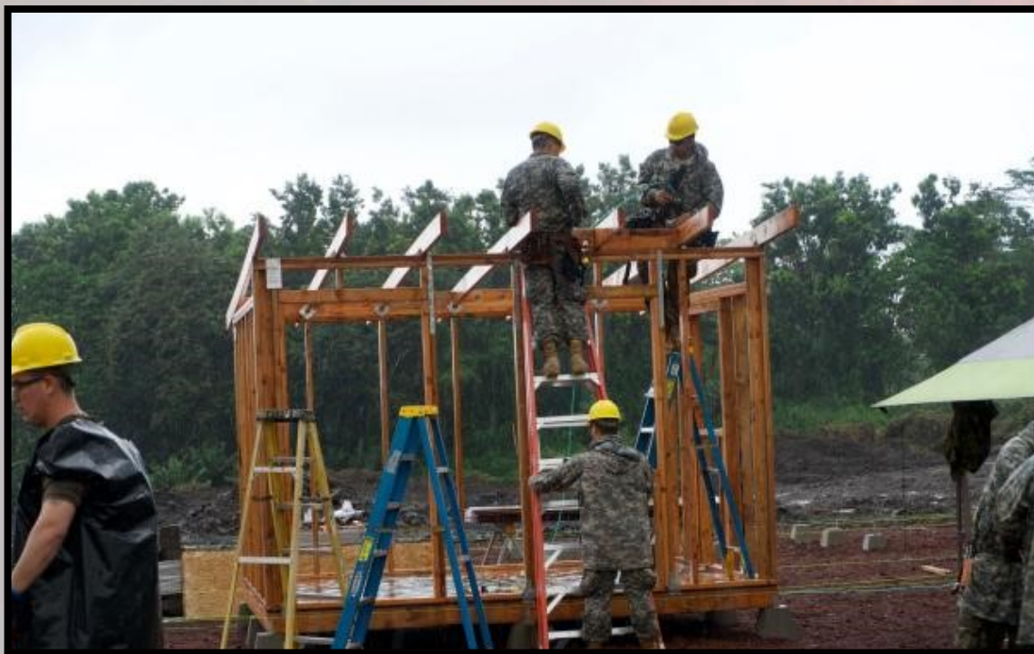
Soldiers from the 230th Vertical Engineer Company, Hawaii Army National Guard, work on the wood framings of one of the twenty shelters that will to be built in Pahoehoe, Hawaii, June 7, 2018. To Date, more than 600 homes have been destroyed by the lava flow. Service members from the Hawaii National Guard teamed up with local organizations to help build micro-shelters for the displaced residents affected by the Puna lava flow. (U.S. Air Force photo by Staff Sgt. James Ro)
